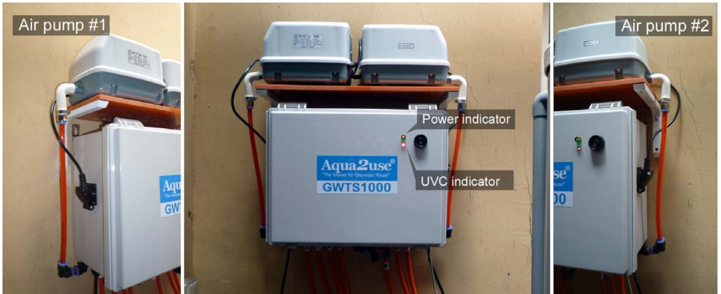
Figure 4. Control box installation
